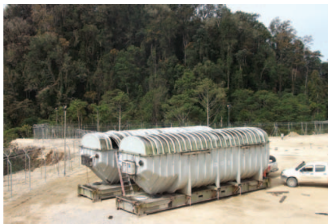
Plate 9.3 – Wastewater treatment plants ready for installation at Paua Camp 6
