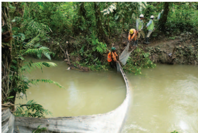
Plate 11.1 – Installation of silt curtains downstream of the Ai’io River crossing
