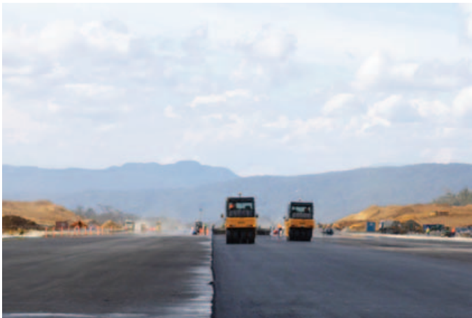
Plate 2.2 – The final asphalt layer on a section of the runway
