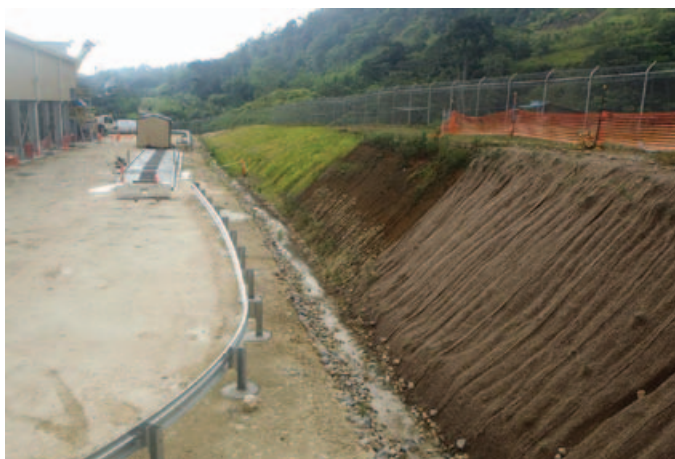
Plate 11.2 – Seeding and jute mesh at the Hides Waste Management Facility process building
