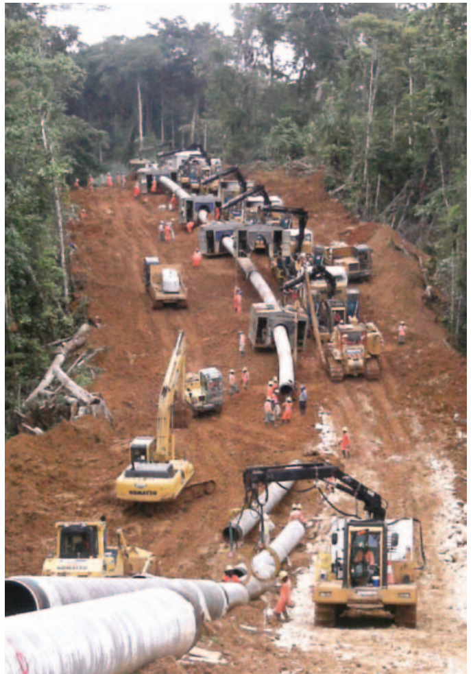
Plate 2.4 – Mainline welding at Kilometre Point 103
