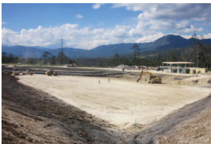
Plate 9.2 – Installation of landfill limestone base at the Hides Waste Management Facility
