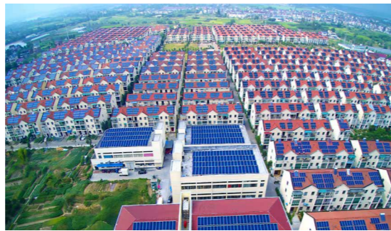
Chint Energy's distributed PV power station project
