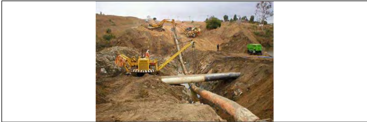
Figure 4. Open-cut river crossing, horizontal flume pipes above pipeline for water flow 12
