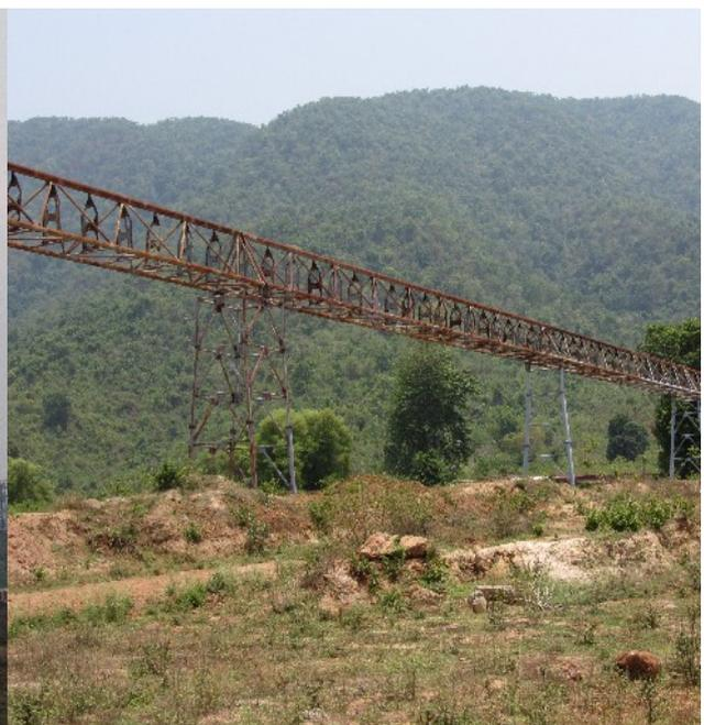
The conveyor belt to carry bauxite from the hill
