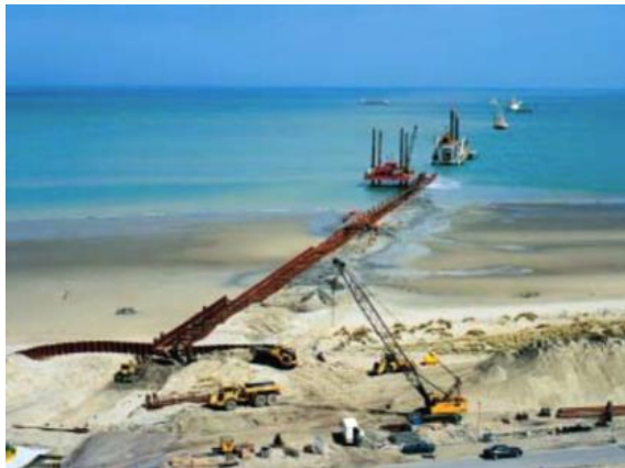
A. Typical shore crossing using sheet piling. Photo: Jan De Nul Group.
