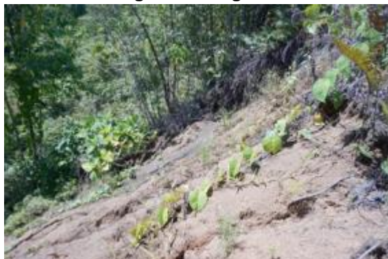
Plate 7.72 – Landslip on a Sidecast Slope Showing Failed Regeneration
