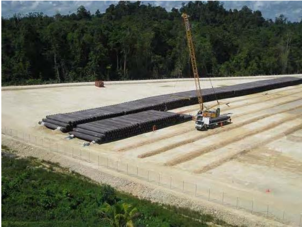
Plate 4.6 – Typical Pipe Yard Laydown Area
