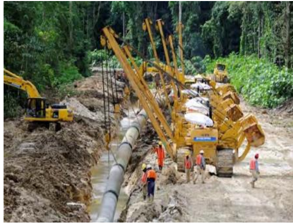
B. Pipeline laying spread. Photo: TOTAL.
