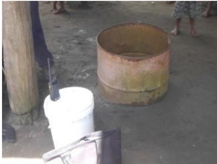
Plate 7.7 – Well With Steel Drum Used for Casing
