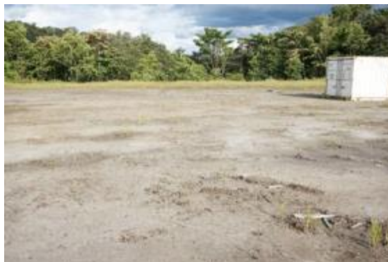
Plate 7.73 – Bare Hardpack on a Wellpad Surface
