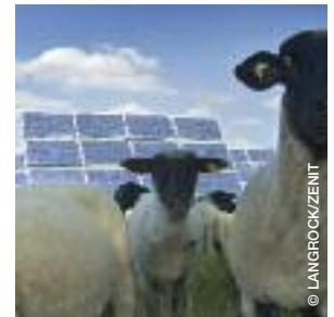
image Photovoltaics facility at 'Wissenschafts und Technologiezentrum Adlershof' near Berlin, Germany. Sheep between the 'movers' keeping the grass short.
