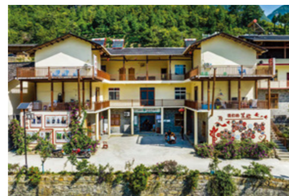
"Xiazhuang Sky Road" homestay upgraded and renovated by villagers
