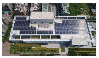
Figure: The Education Building in Wuri, Taichung has installed solar panels (183 kW) and received the LEED Gold Certification.
