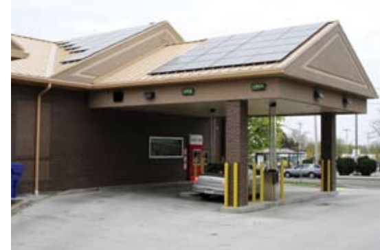
This HSBC branch in Greece, New York, has solar panels on its roof – an example of renewable energy technology trialled by HSBC.
