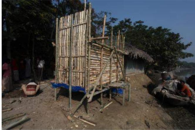
**Figure 5.** Joymoni -Interim Oil Impacted Debris Storage and dewatering photodocumented on 23 Dec by Kawser Mohammad, UNDP
