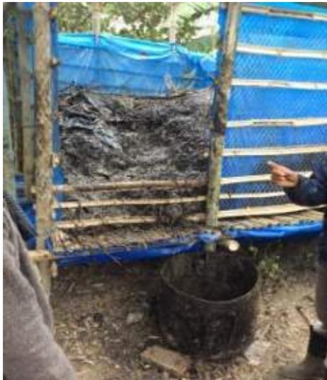
**Figure 6.** Joymoni Residence - Interim Oil Impacted Debris Storage and Dewatering Crib photodocumented on 27 Dec by Keith Donohue UNDP
