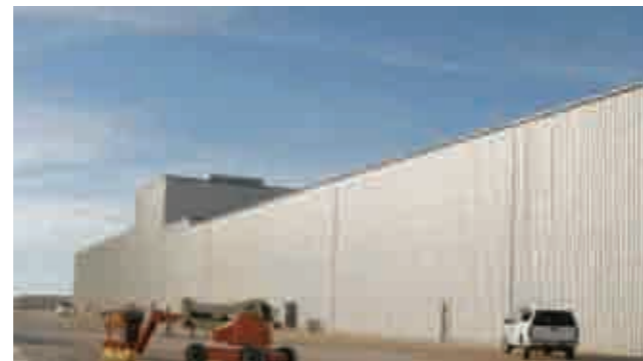
The Centrifuge Assembly Building - handed over to ET US in late October 2008
