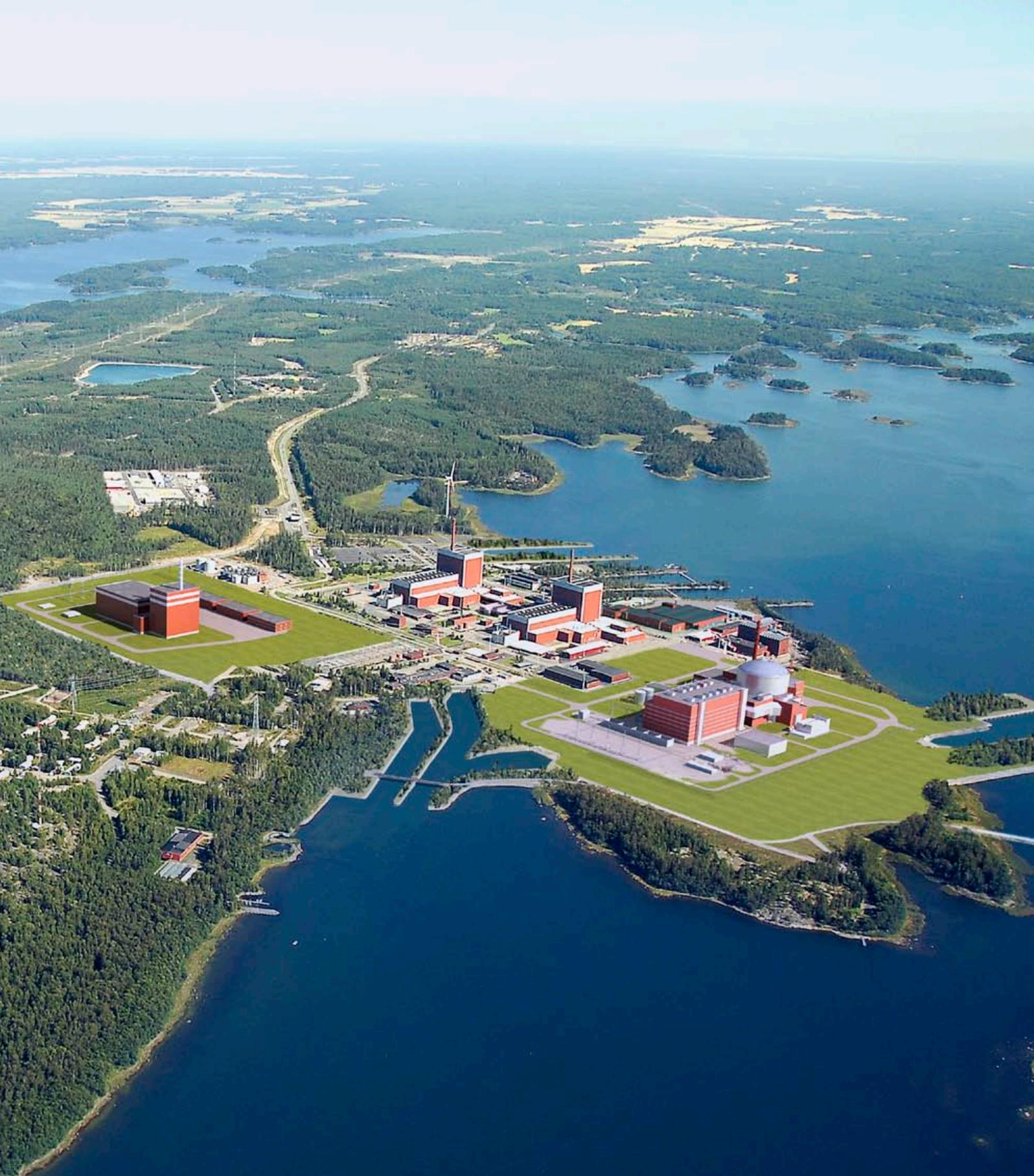
*In the middle: the operating OL1 and OL2 units on the western shore of Olkiluoto Island. The OL1 unit has been generating electricity for more than 30 years. To the right: photo montage of the OL3 nuclear power plant unit now under construction.*
