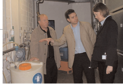
Inspection of the waste water facility at Deutsche Bank’s headquarters.
