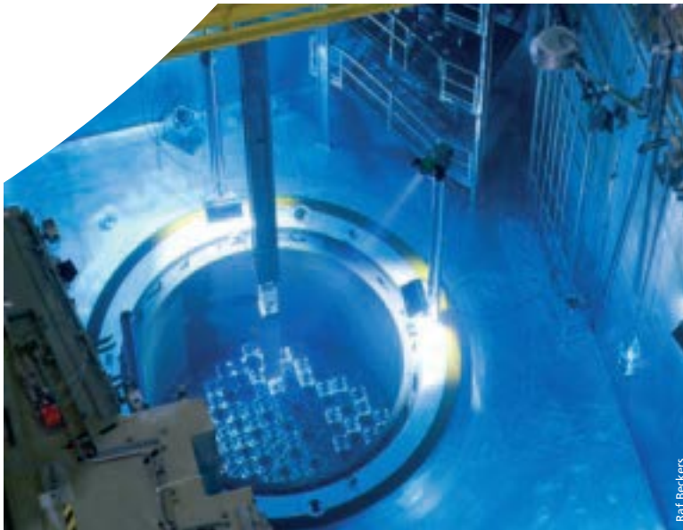
Reactor vessel reloading
