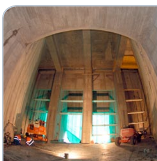
The cooling water intake tunnel has a cross-section of about 60 \text{ m}^2 .
