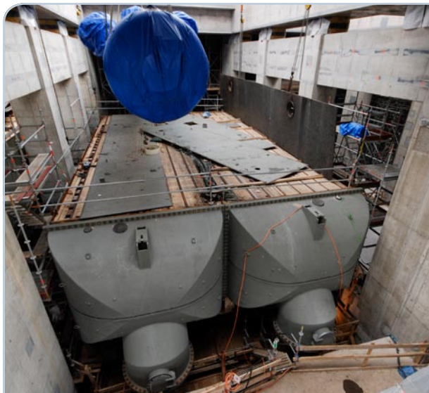
Sea water chambers in condenser unit installed in place.
