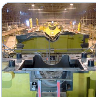
Turbine bearing structures being installed at the turbine hall floor level. The bearing pedestals are being aligned and installed on the turbine foundation.
