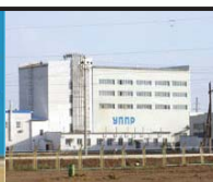
Processing Plant, Akdala
