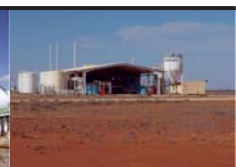
Demonstration Plant, Honeymoon
