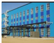
Processing Facility, South Inkai
