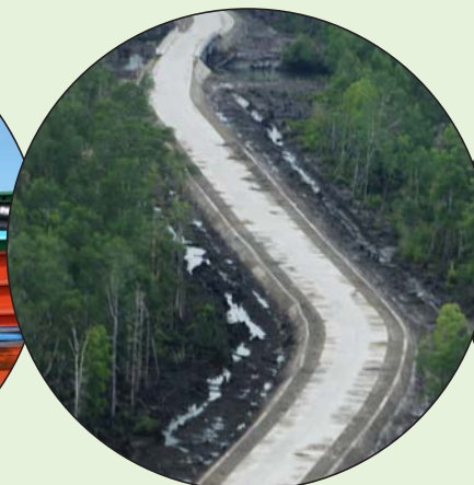
A portion of a new road paved with tailings in Papua
