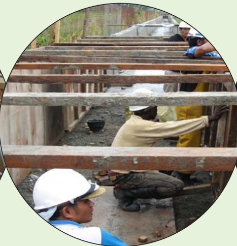
CV Bulbuk Activities Mozes Kilangin Airport
