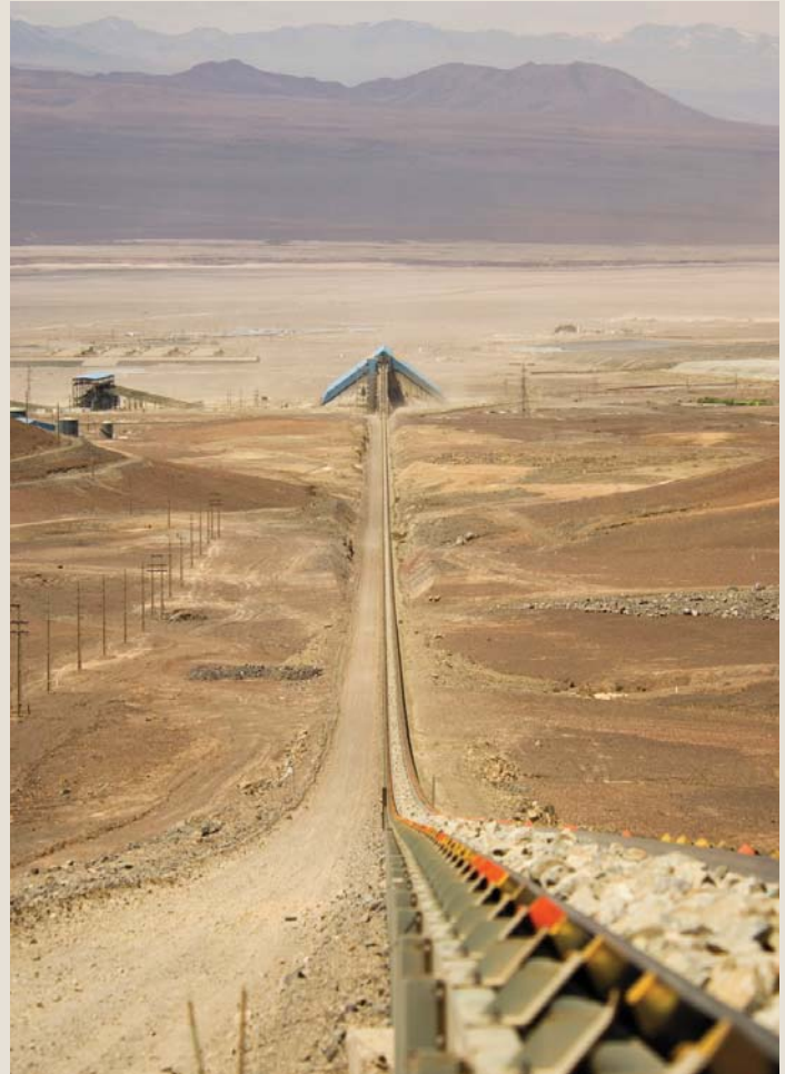
This conveyor belt presently in use today to carry ore for further processing will continue to be used in the future sulfide project.
