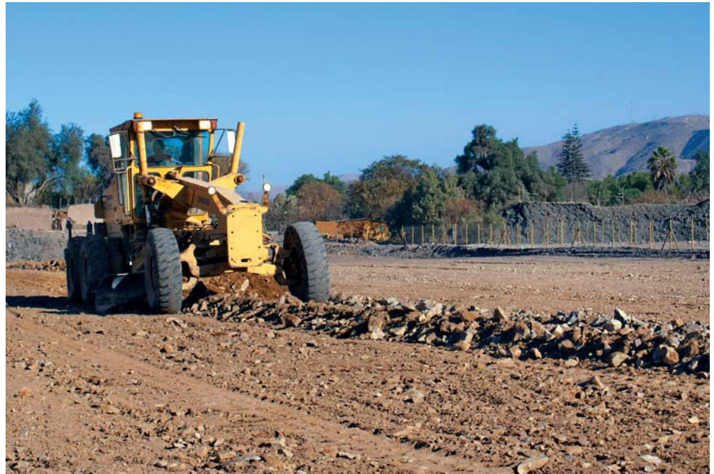
Cleanup underway to remove slag and refuse.
