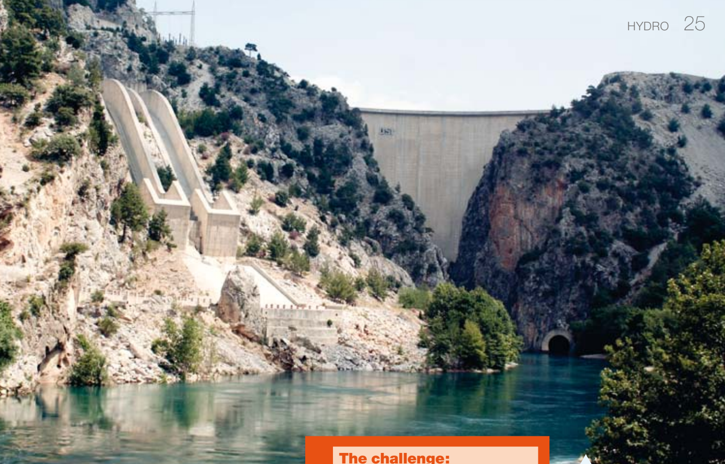
Gentle hydropower: Oymapinar pumped storage power station, Turkey.
