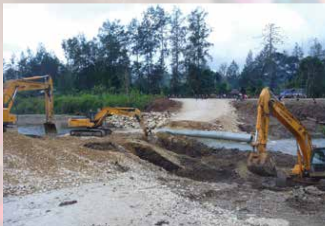
Work underway on the road outside Tari 2011. Photo credit: James McIlraith/ University of Otago
